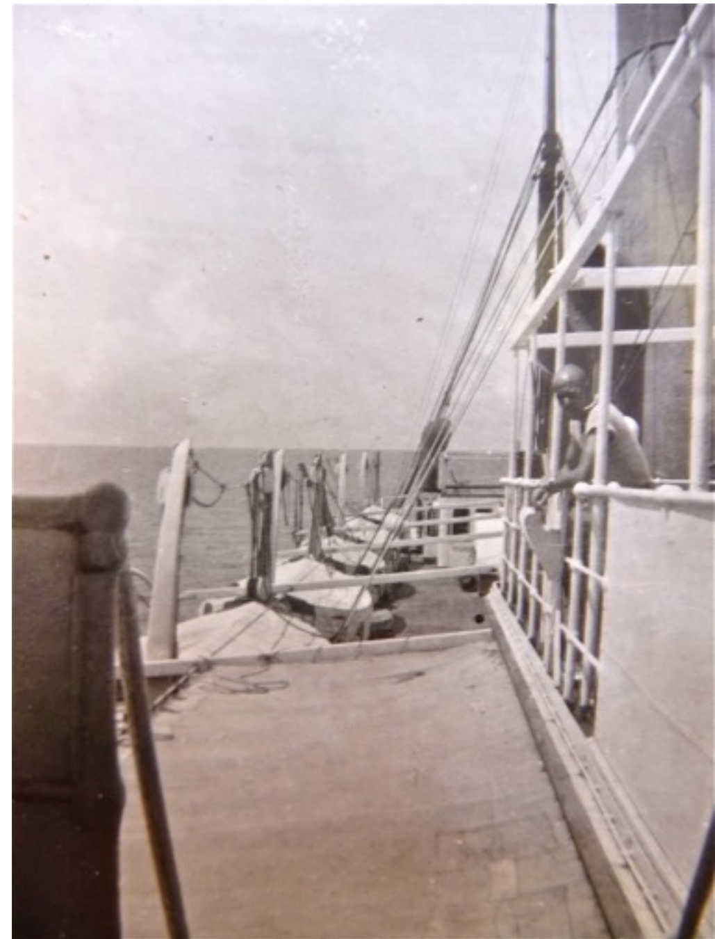
Best Overend. On the side of the Bridge.
