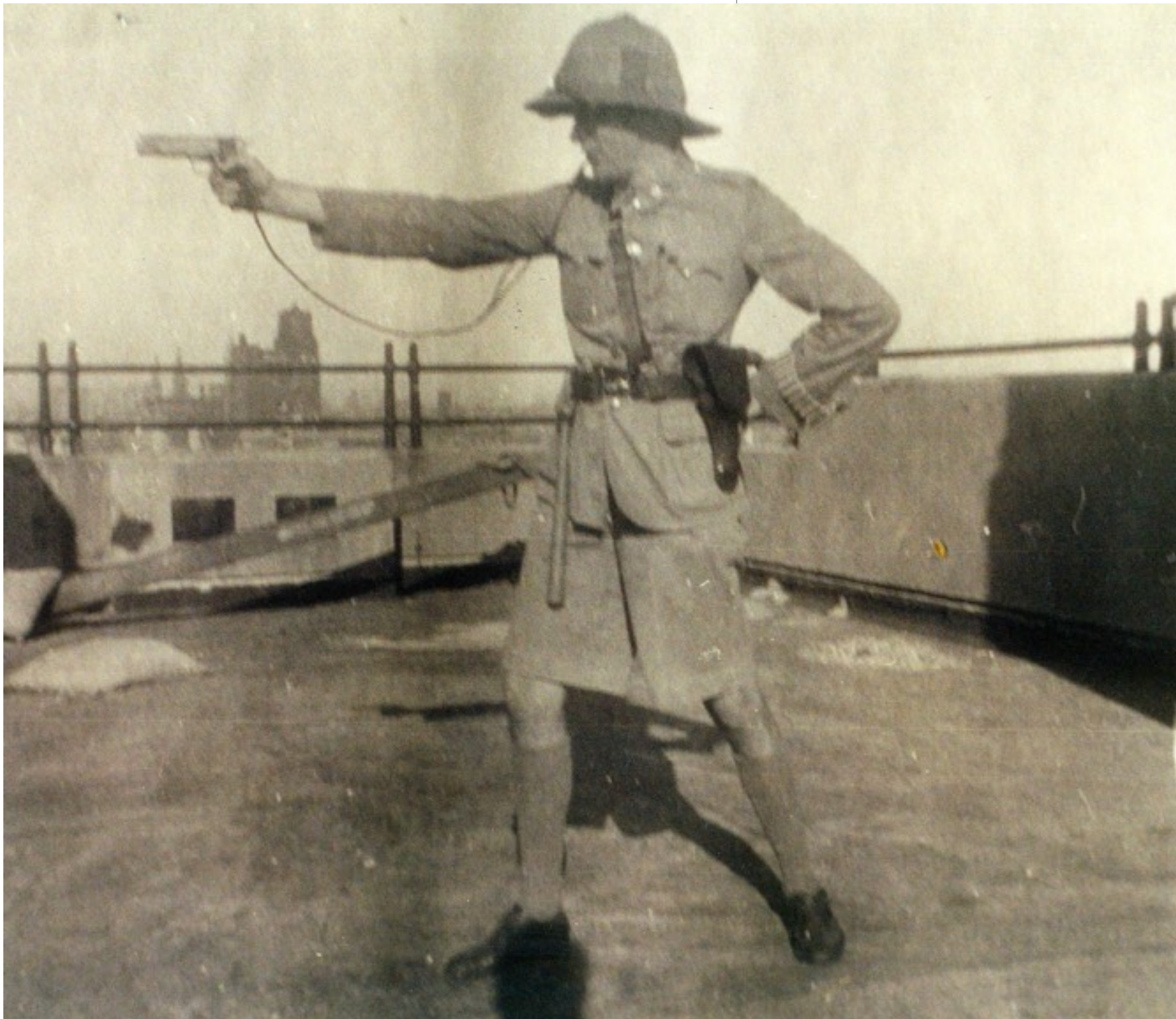
Roof top pose. Best Overend in the uniform of the Shanghai International Police Force, complete with baton and drawn .45 Mauser. The eight story building , on the Bund, was having a new flat roof installed by his employer, the Architectural practice, Lester, Johnson and Morriss.
